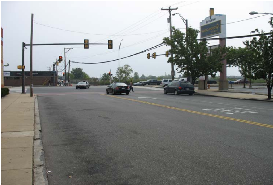
Figure 1: Overhead utility along Reed Street at Columbus Blvd.
