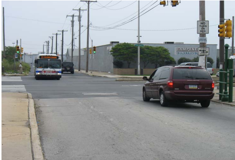
Figure 3: Insufficient turning radii on curbs at Columbus Blvd. and Tasker Street
