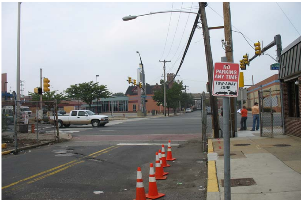
Figure 2: Insufficient turning radii on curbs at Columbus Blvd. and Reed Street
