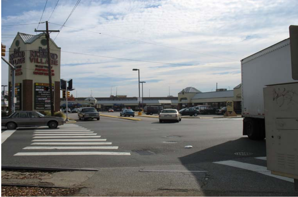
Figure 2: Missing pavement markings at Port Richmond Village Shopping Center exit
