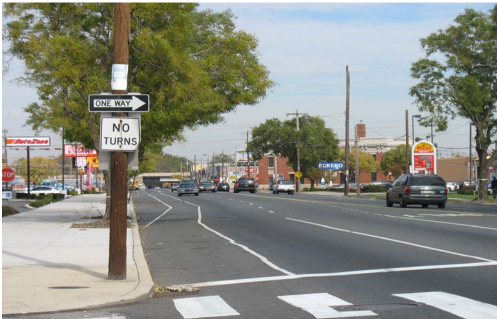
Figure 3: Bike lane used as right turn lane at Cumberland Street and Aramingo Avenue intersection
