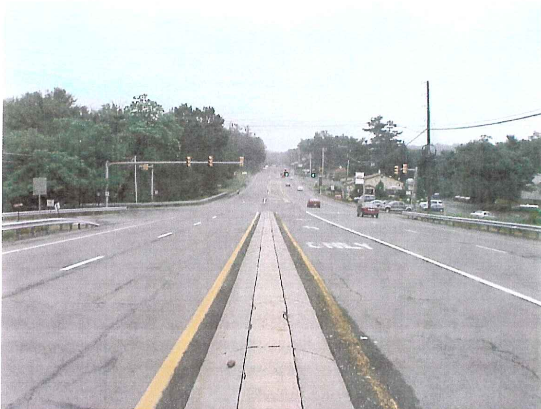
Direction / Road: Southbound Route 611 Approach / Departure: Approaching Woodland Road
