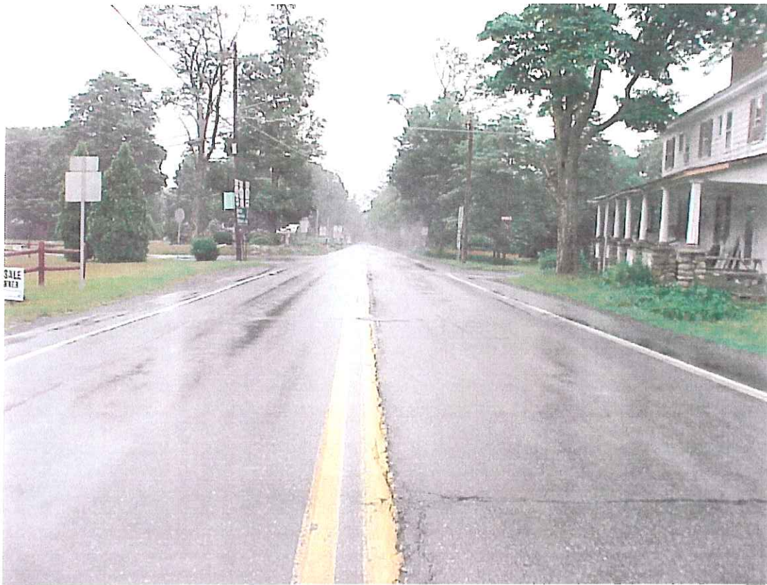
Direction / Road: Eastbound Route 940 Approach / Departure: Approaching Route 191/Red Rock Road
