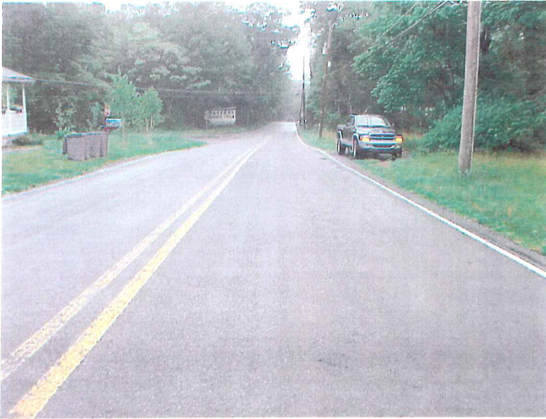
Direction / Road: Northbound Carlton Road Approach / Departure: Approaching Woodland Road
