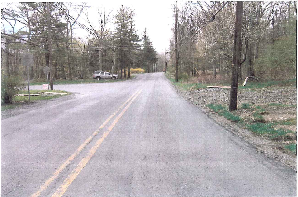
Direction / Road: Westbound Woodland Road Approach / Departure: Approaching School Driveway
