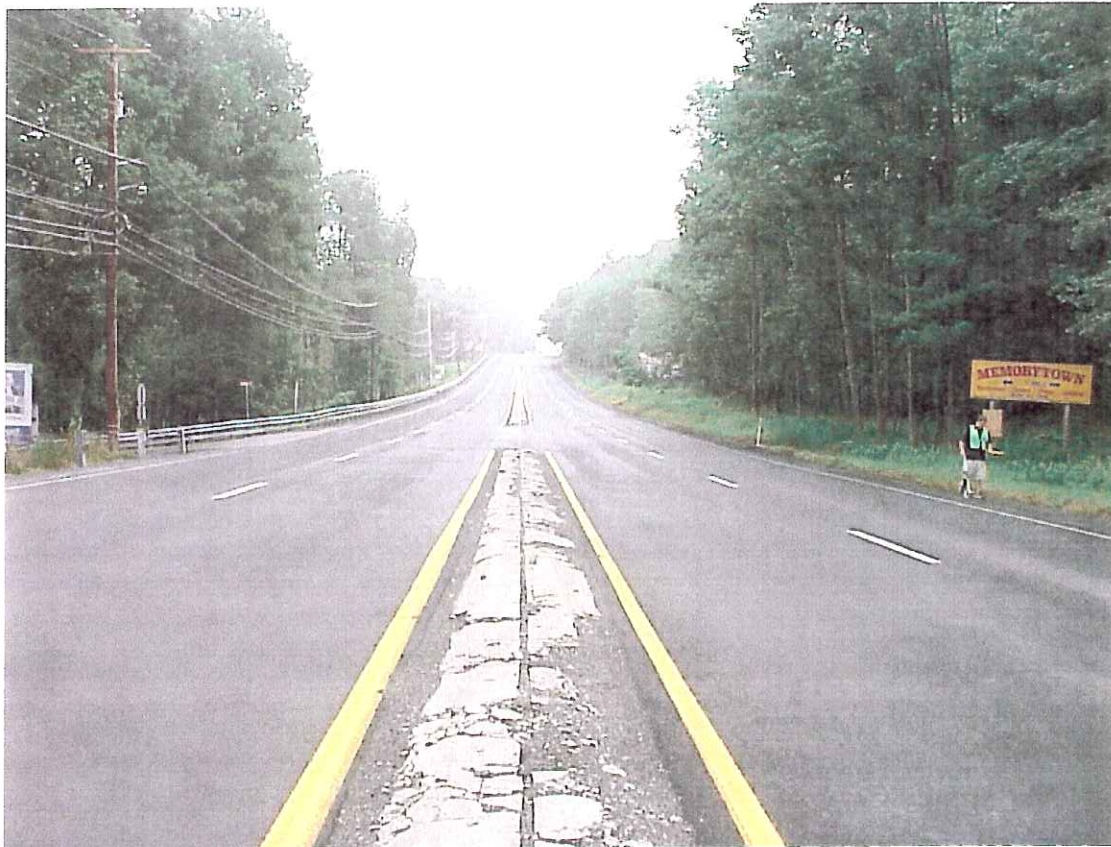
Direction / Road: Southbound Route 611 Approach / Departure: Approaching Grange Road
