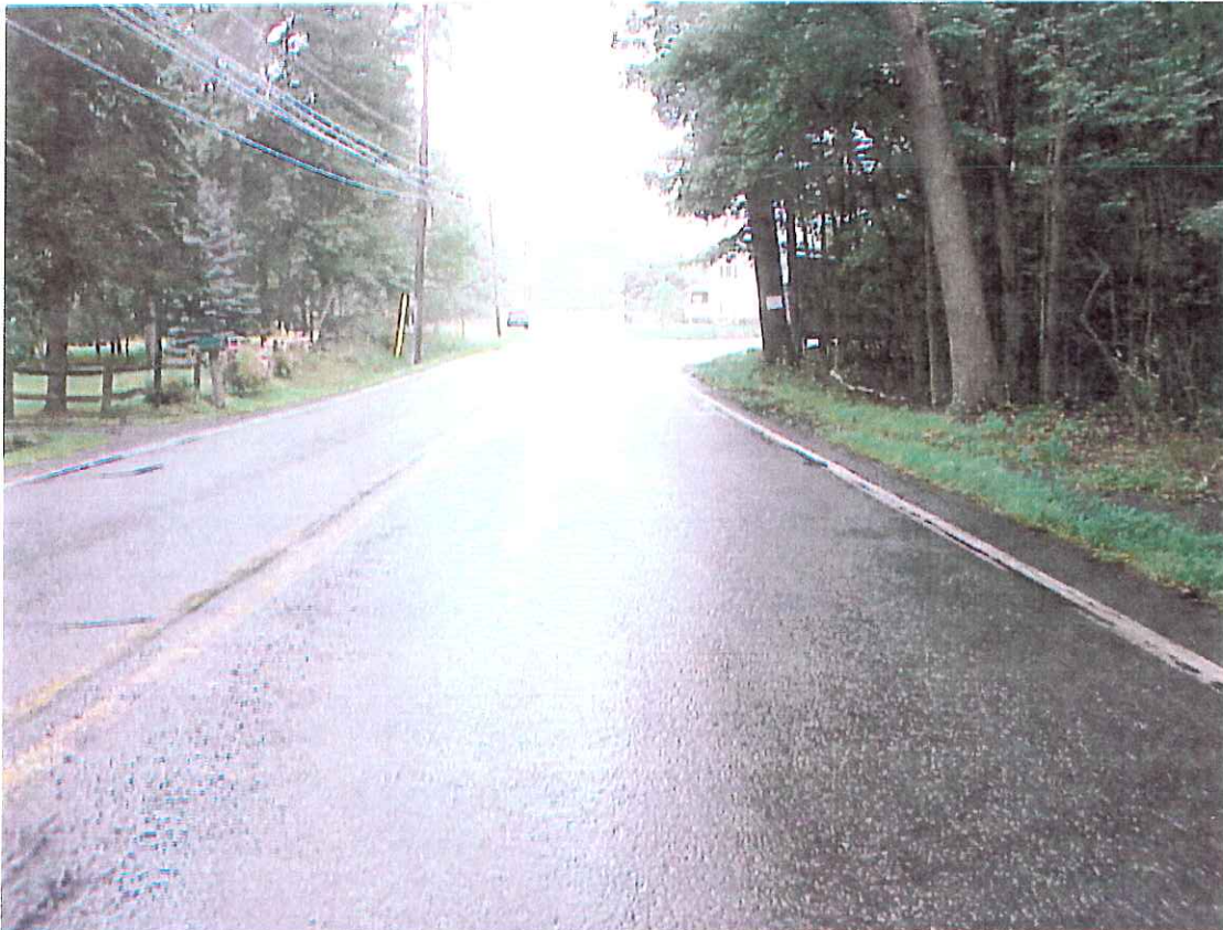
Direction / Road: Southbound Carlton Road Approach / Departure: Approaching Woodland Road
