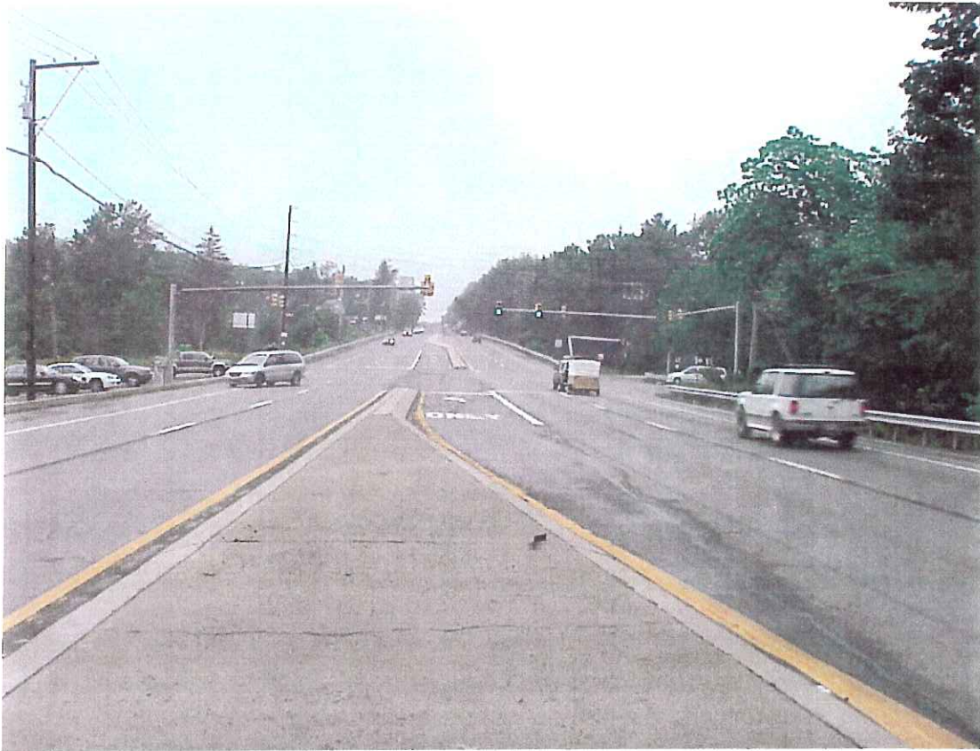
Direction / Road: Northbound Route 611 Approach / Departure: Approaching Woodland Road
