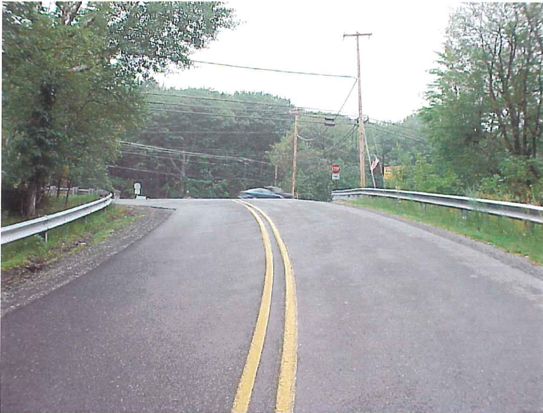
Direction / Road: Westbound Meadowside Road Approach / Departure: Approaching Route 611
