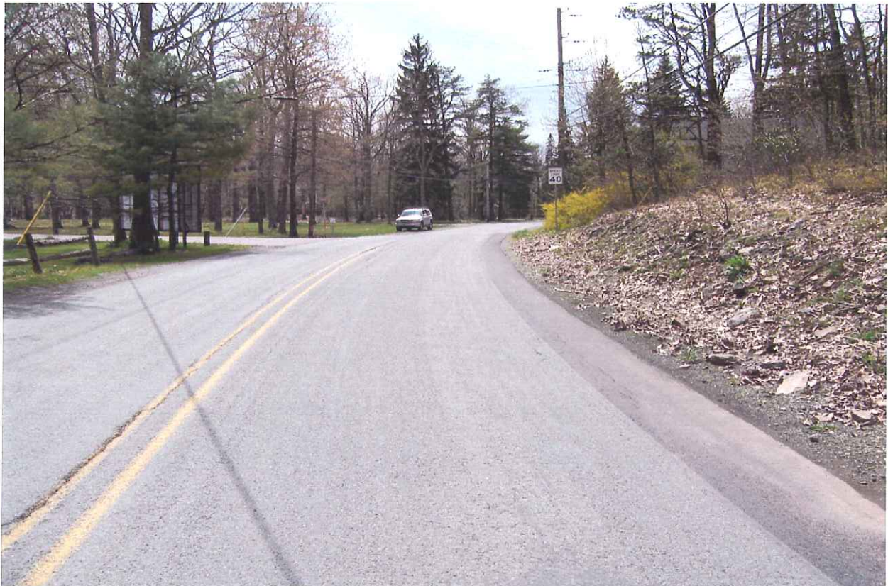
Direction / Road: Westbound Bowman Road Approach / Departure: Approaching Woodland Road
