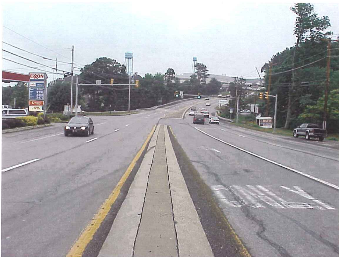
Direction / Road: Southbound Route 611 Approach / Departure: Approaching Route 314
