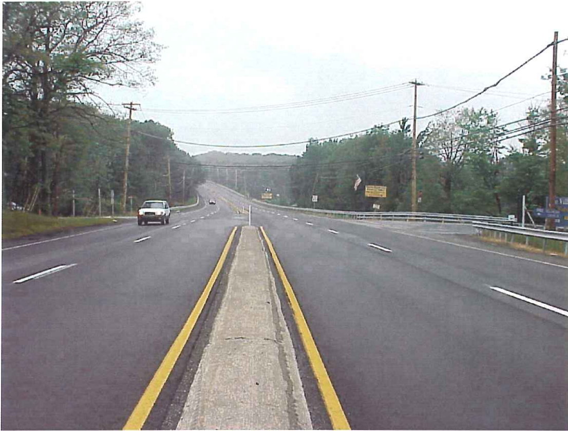
Direction / Road: Northbound Route 611
