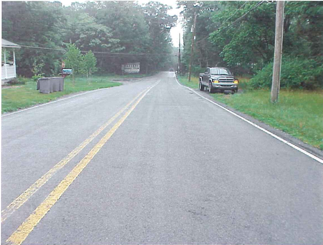
Direction / Road: Northbound Carlton Road Approach / Departure: Approaching Woodland Road
