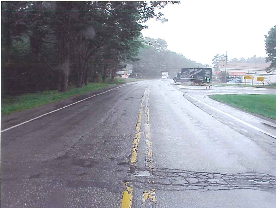
Direction / Road: Westbound Route 940 Approach / Departure: Approaching Route 390
