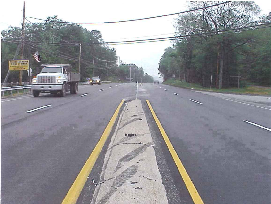
Direction / Road: Southbound Route 611
