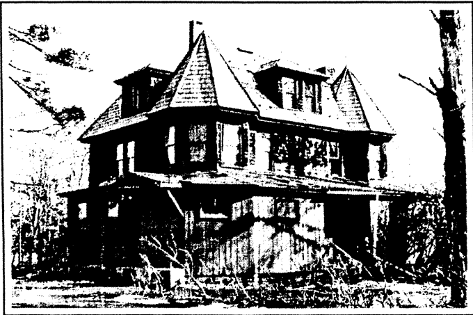
Photograph No. 5 – Late Victorian cottage, looking southeast. This is one of the properties of Strickland's Mountain Resort.
