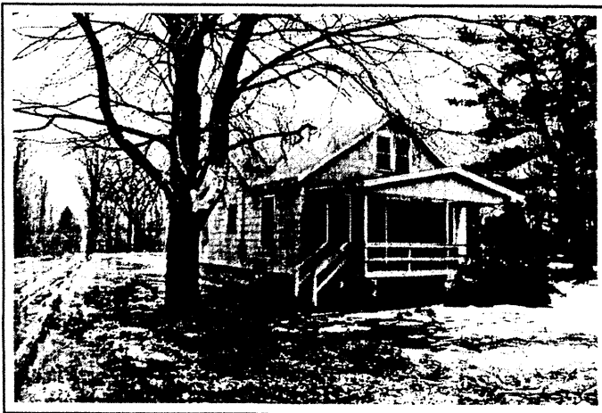
Photograph No. 3 – A circa 1930 resort cottage, looking south.
