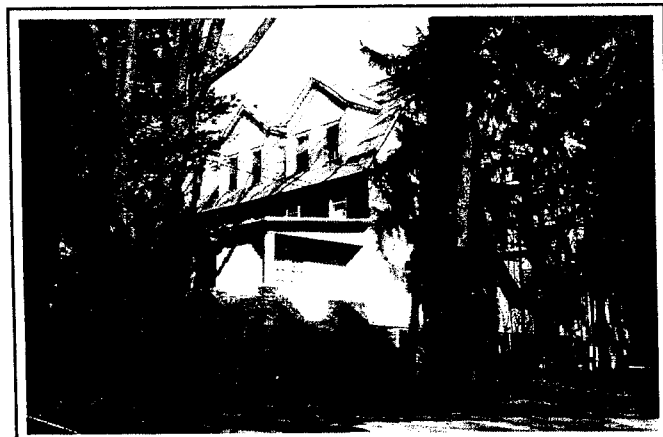
Photograph No. 6 – Original main building of Strickland's Mountain Resort, looking northeast. The gambrel roof and gable-end dormers suggest a date of circa 1920.
