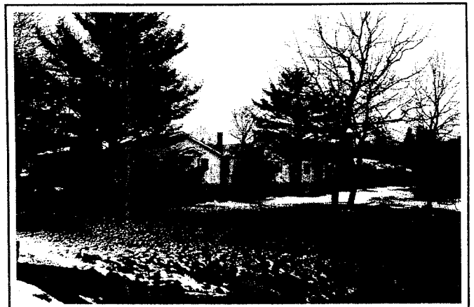
Photograph No. 4 – Circa 1930 resort lodges, looking northwest.
