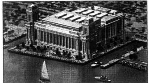
Former electric generating station in Chester, Pa., transformed into an office building.
