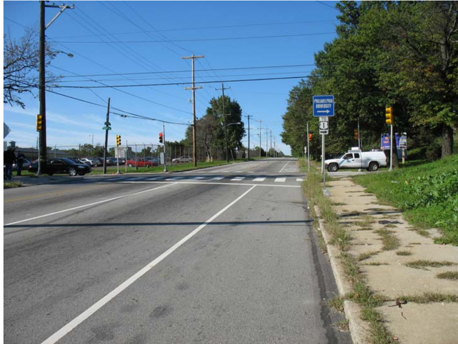
Figure 3: Westbound Roberts Ave. at the intersection of Roberts Ave. and Fox Street
