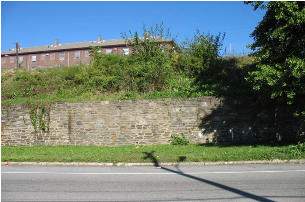
Figure 5: Roberts Ave. near site access – Retaining Wall
