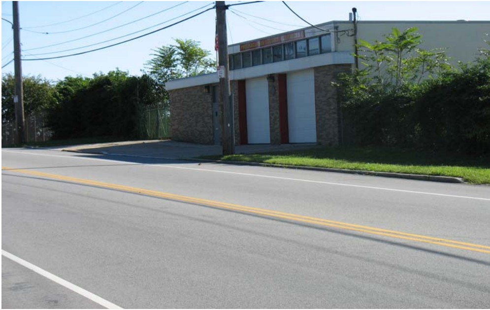
Figure 4: Roberts Ave. near site access – Philadelphia Second Alarmers Fire Station
