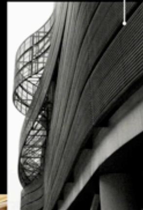
FLOWING INTERIOR SURFACING
