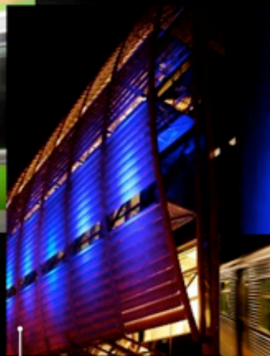
MULTI-LAYERED GARAGE EXTERIOR MEMBRANE
