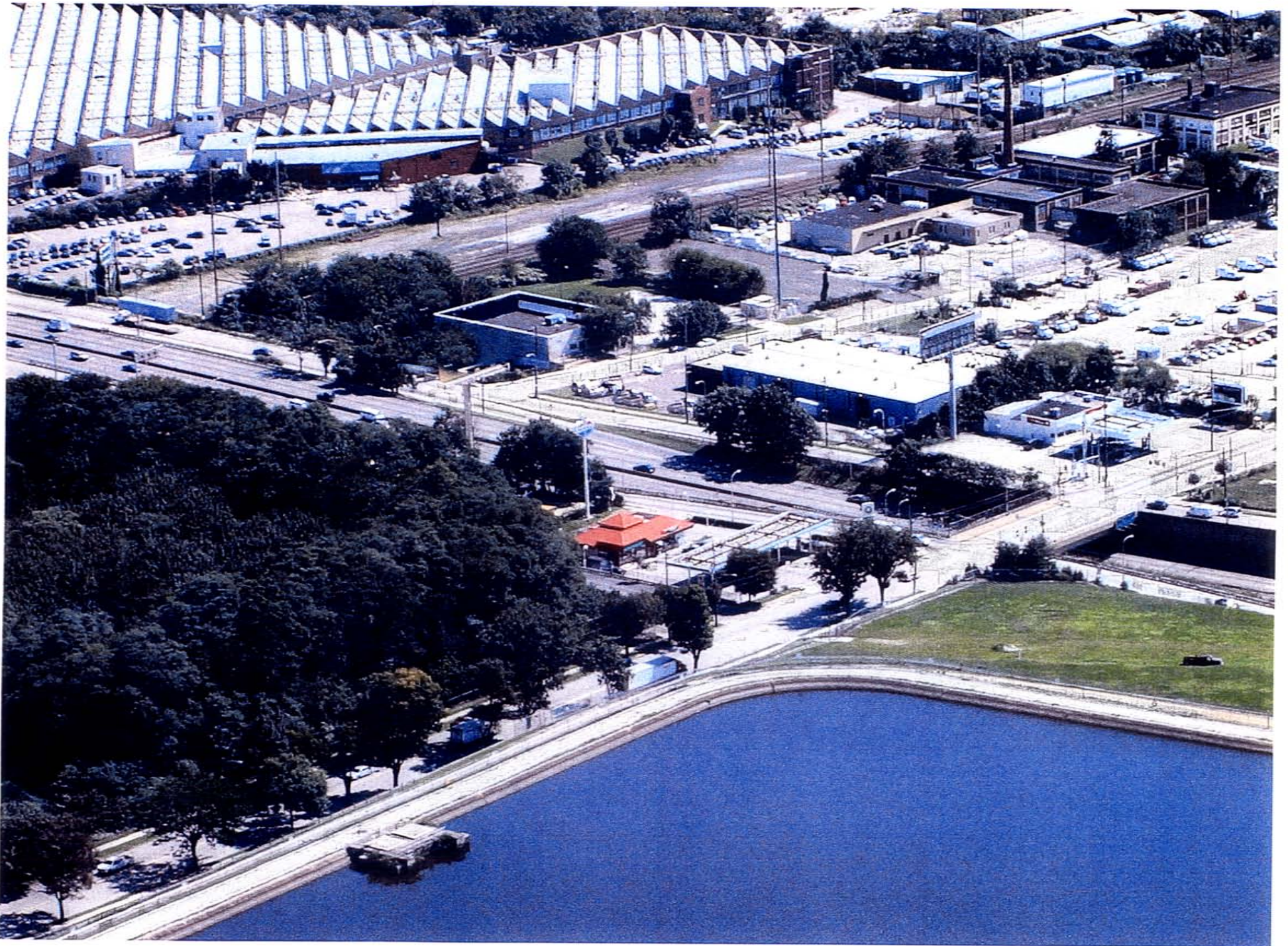
Existing Route 1 Northbound Off-Ramp
