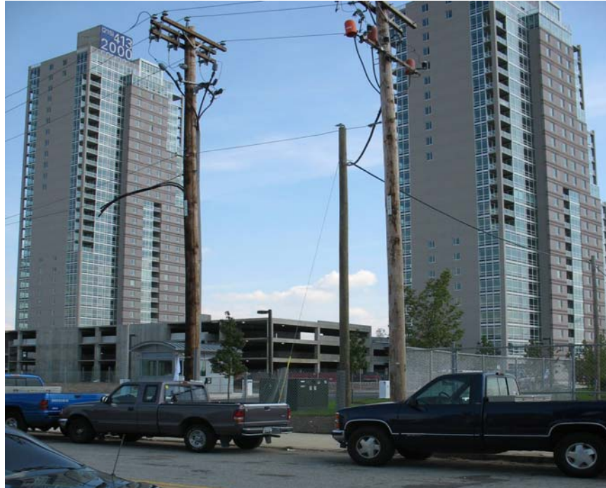
Figure 1: High-rise Condominiums Under Construction on Penn Street
