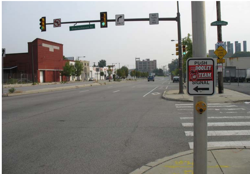
Figure 4: Utilities in the Parking Lane on Delaware Avenue at Shackamaxon Street
