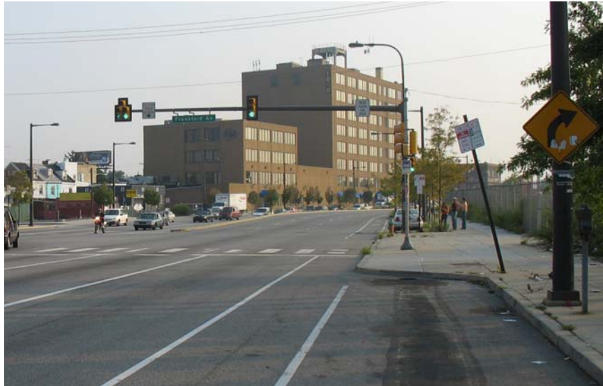
Figure 5: Utilities in the Parking Lane on Delaware Avenue at Frankford Avenue
